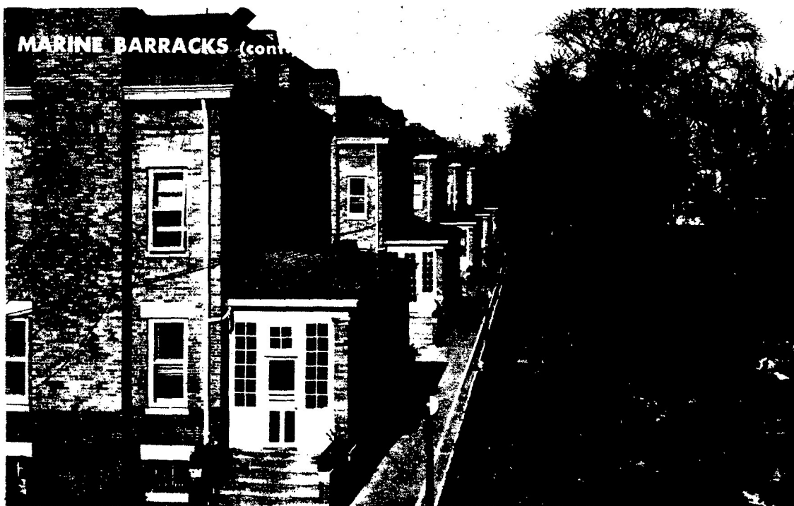
Officers' homes at Eighth and Eye are spacious, modern brick buildings which border one side of the parade ground. Some believe this part of the compound was the site of old Center House
